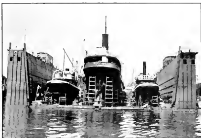
The smaller section of the Wallace Dry Dock at Vancouver with the steamship Prince John and two tugs up.
